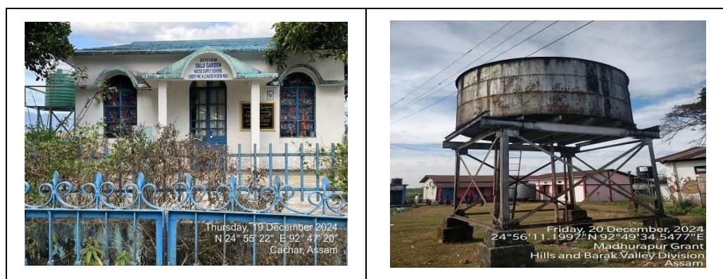
Figure 3-29: Drinking Water Facilities in the study area
