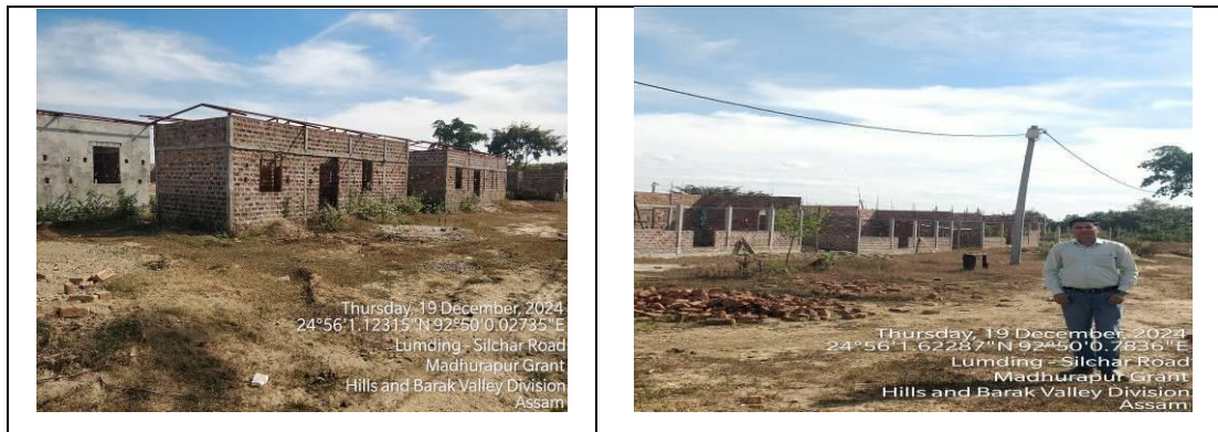
Figure 3-33: Houses under construction at Rehabilitation Site
